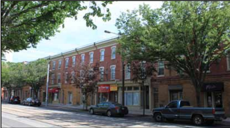
3600 block of Lancaster Avenue, aka Lancaster Mews. Photo by Joseph Minardi.
