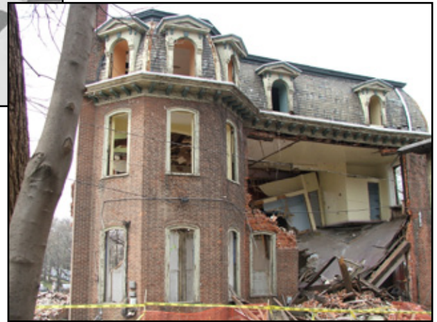
Demolished c. 1860 mansion that stood on the site of the proposed 4224 Baltimore Avenue. Photo by Melani Lamond.
